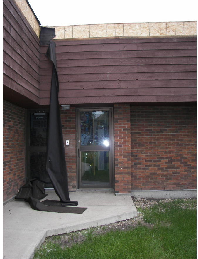
(1978) Metal flashing is being installed on site.
