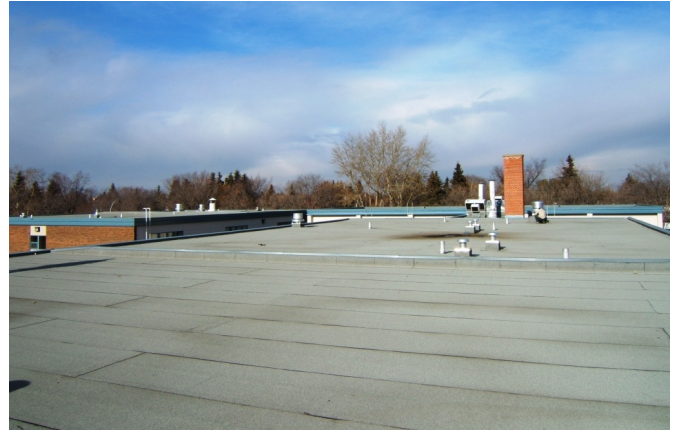
View of 1958 Roof Section.
