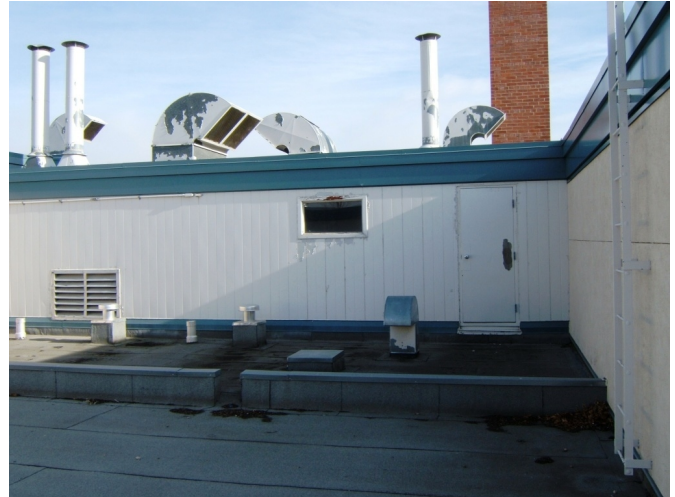
Painted mechanical room exterior finish.
