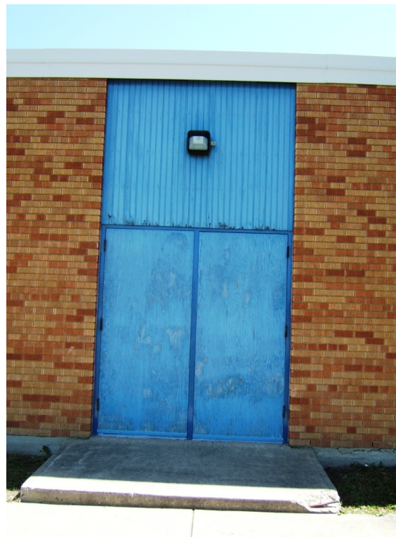
Painted wood panels over exterior doors.
