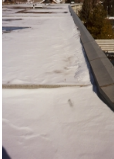
Roof Parapet at East Façade
