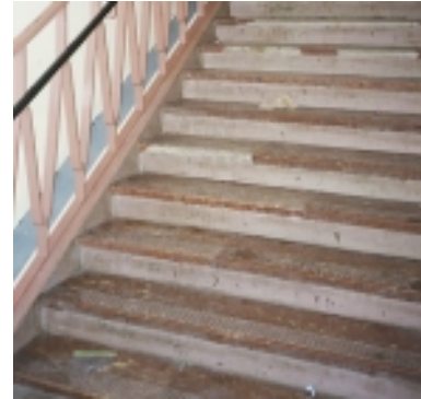
Typical Condition of Stairwells
