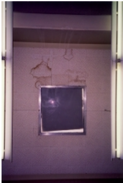
Leaking Skylight
