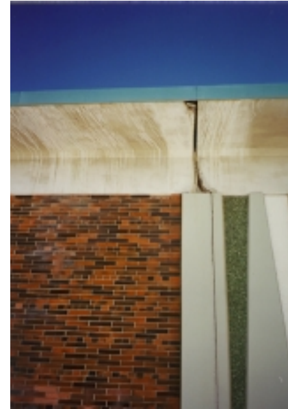
Roof Tees at Column Location
