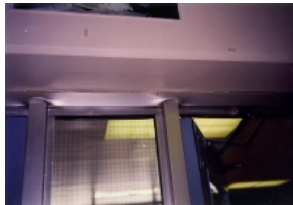
Detail - Compressed Door Frame
