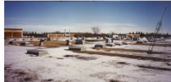
Industrial Arts Roof
