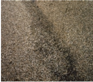
Heaving Roof Membrane at Industrial Arts
