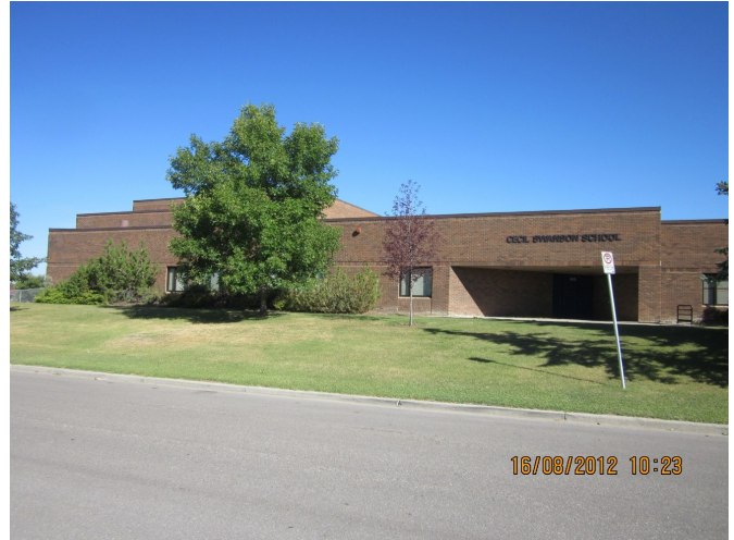
View of west front of school
