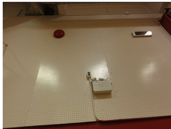
Aged emergency lighting battery unit is not plugged in. Heads are not aligned properly.
