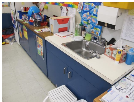
Original millwork in classroom area.
