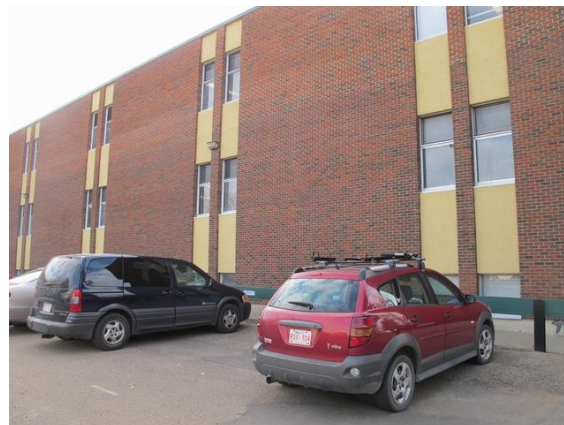
Original 1972 and 1968 Windows
