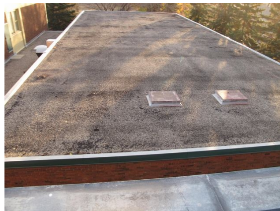
Original roof above 1963 Section
