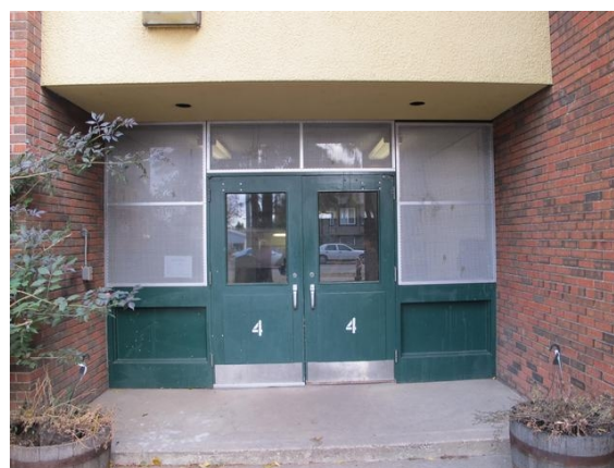
Main entrance doors - South elevation
