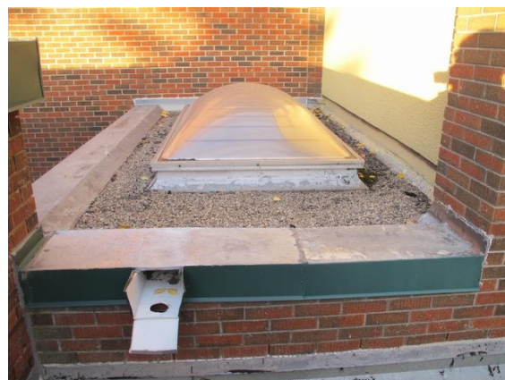
Skylight above stairwell in 1972 Addition
