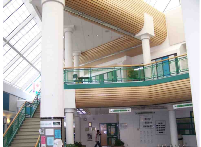
Wood handrails with painted pipe support and painted metal mesh inlay sections.
