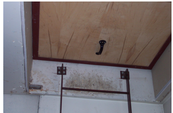
Plywood hatch from Storage Room 010 to Mechanical Room 102
