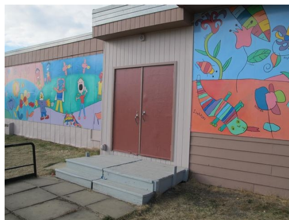
Exit doors at east link
