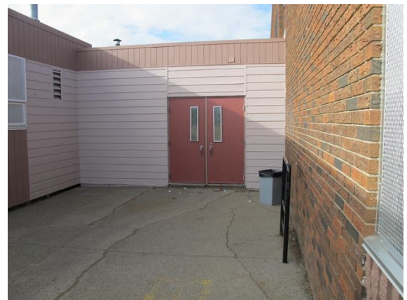
Exterior exit doors - South Link - North entry
