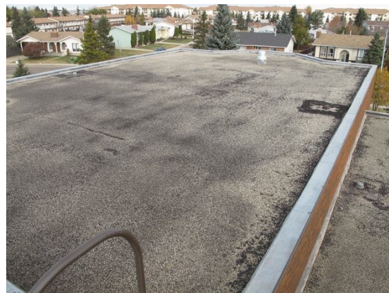
Typical condition of the original 1978 Roof
