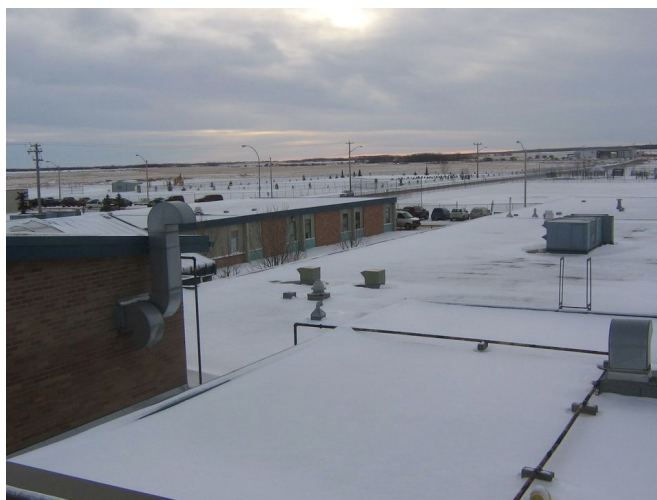
Rusting gas lines on roof.
