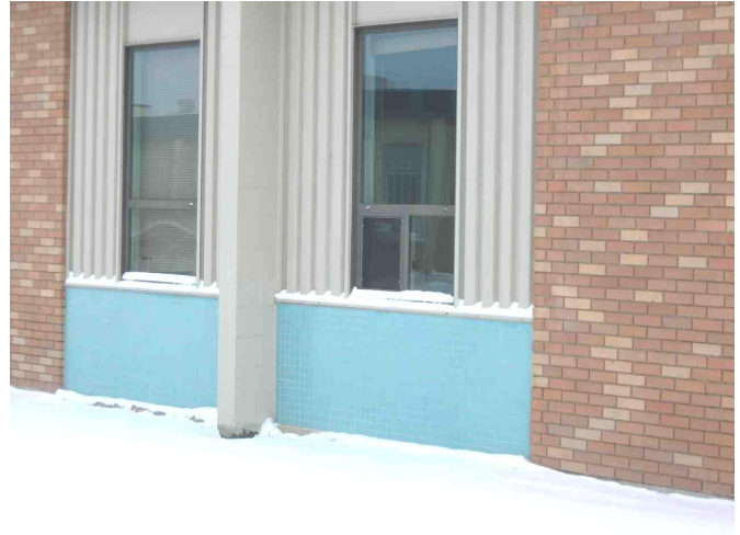
Ceramic tiles under windows and vertical metal siding highlights; 1964 building.
